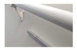
10. Secure the channel into the clips.
