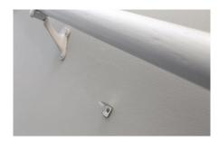
9. Use a ruler to place the mounting clips (included) near the location of the ends of the channels.
